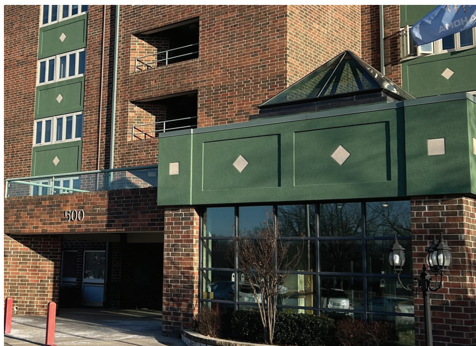
Autumn House in Midwest City is an independent living center for people age 62 and older.
